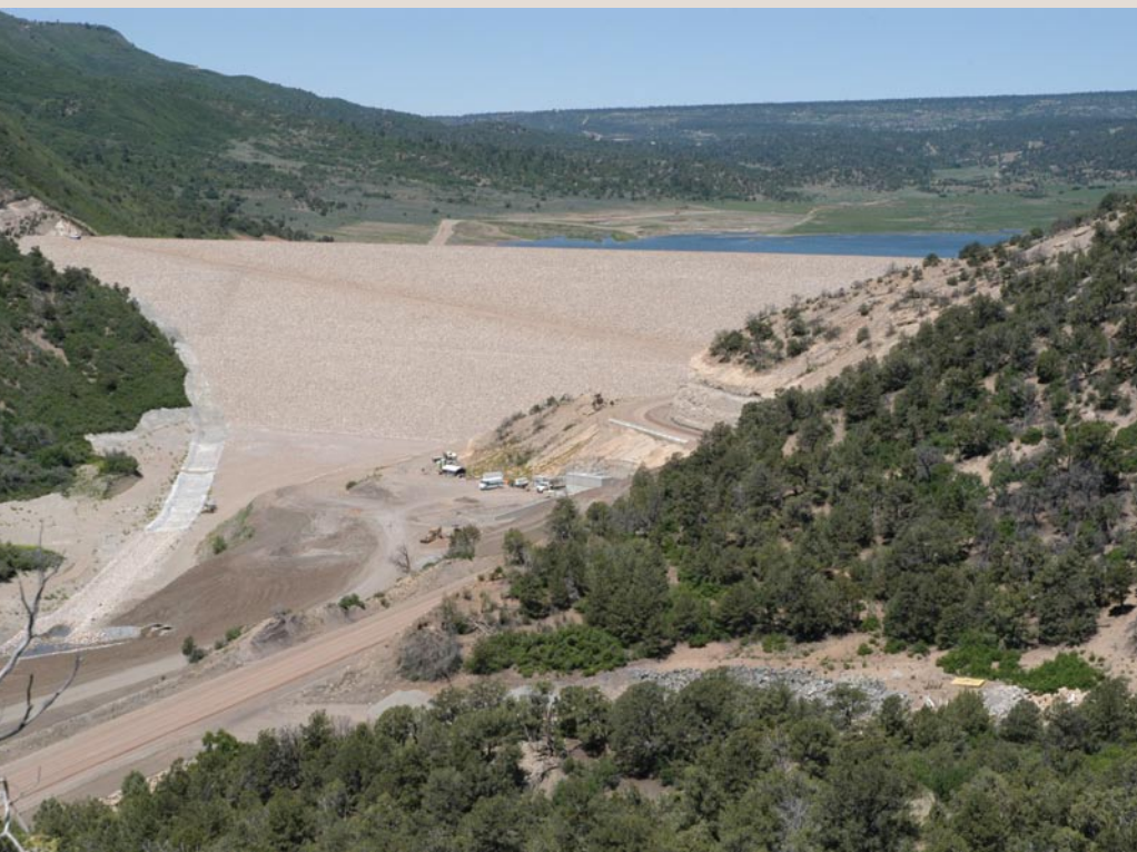
The completed Ridges Basin Dam contained 1,000 acre-feet of water from winter snow melt in July 2008.
