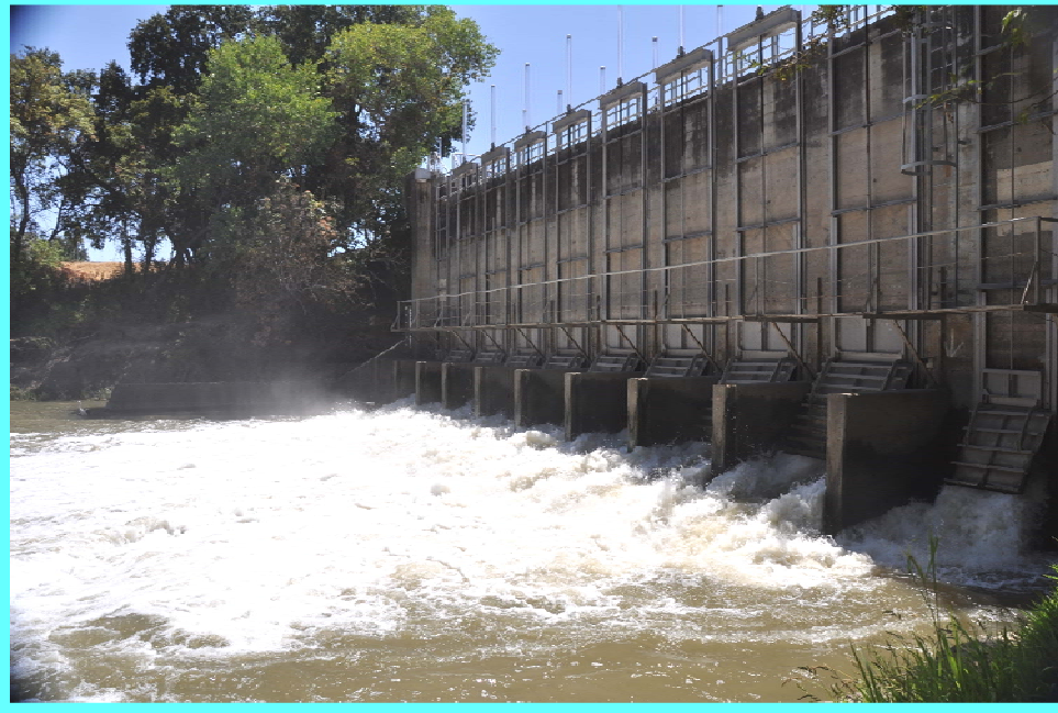
Colusa Basin Drain Outfall Gates
