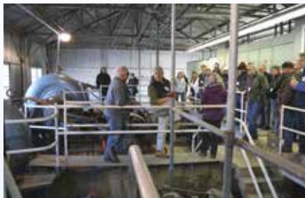
Farmers Tom Slater and Steve Heringer talk about infrastructure and issues in the Sacramento-San Joaquin Delta with participants of our one-day Delta Tour during a stop at Reclamation District 999's pump house.
